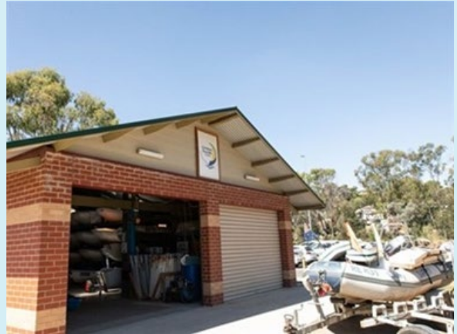
Image description: Red brick structure (boat shed), with open roller door.
