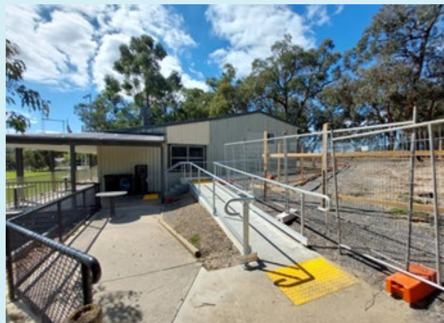
Image description: A new external ramp alongside construction fencing at Narre Warren East Pavilion.
